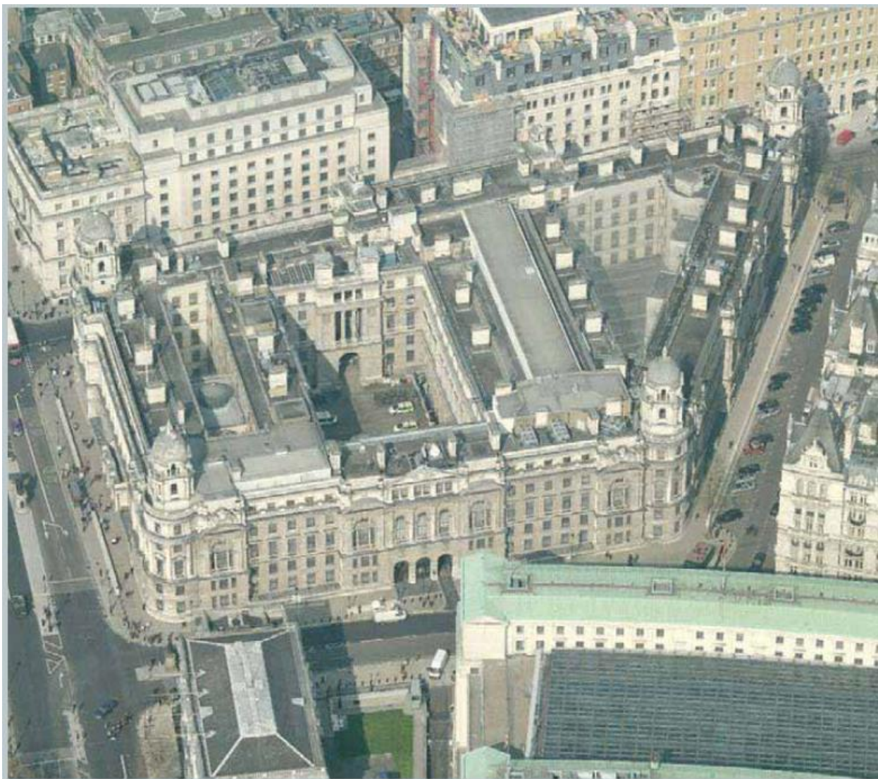
Aerial view of the Old War Office, 57 Whitehall
